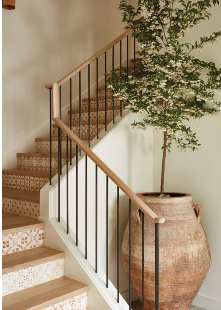
European white oak plank treads from Montello Design with custom handrails and balusters are jaunty. The tile by Tabarka Studio via Ann Sacks on the staircase bring a soft sophistication to each step.
