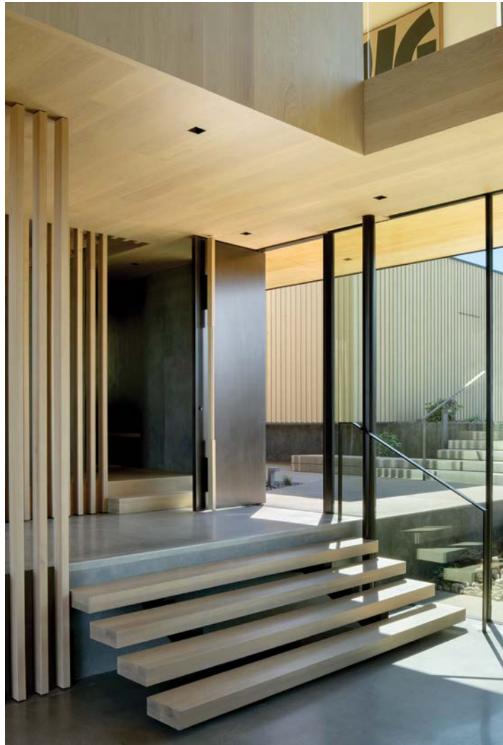
LEFT Blackened steel pivot door from Flux Design with white oak handle is carved midway to perfectly fit a hand. KN Visions cantilevered the hollow boxed entry stair treads without using fasteners. The detached garage opposite the main entry includes a studio, bath and storage. RIGHT Steel and wood room separator fashioned by Max Manufacturing with KN Visions. The floor is polished concrete.
