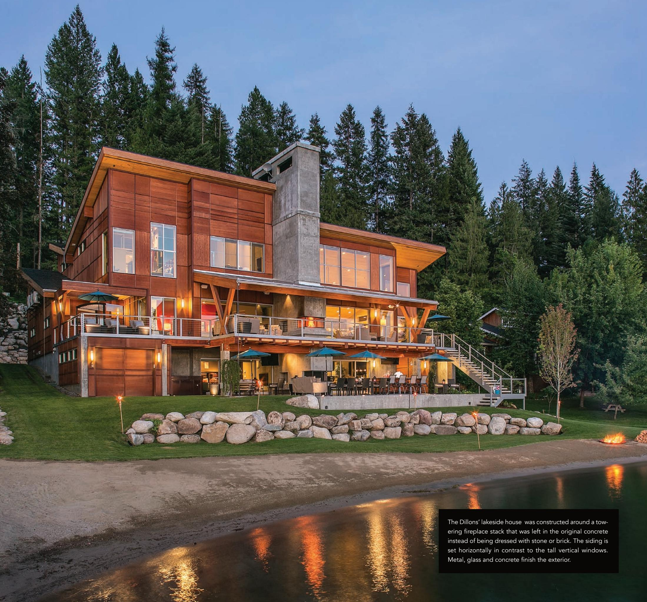
The Dillons' lakeside house was constructed around a towering fireplace stack that was left in the original concrete instead of being dressed with stone or brick. The siding is set horizontally in contrast to the tall vertical windows. Metal, glass and concrete finish the exterior.
